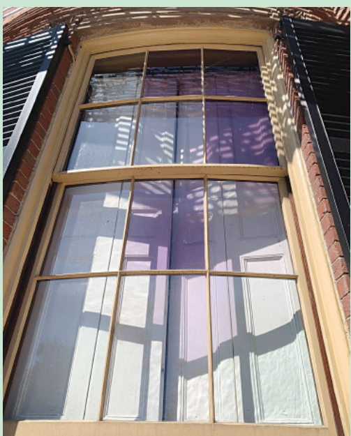
The color of the famous purple windows or “Lavenders” of Beacon Hill was caused by the chemical reaction of manganese oxide to sunlight in the early- to mid-1800s.
