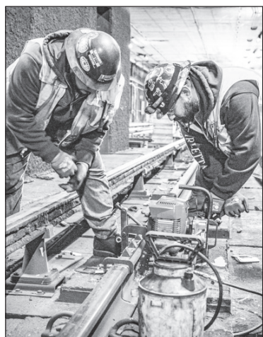
Infrastructure improvements were accomplished along the Red Line.
