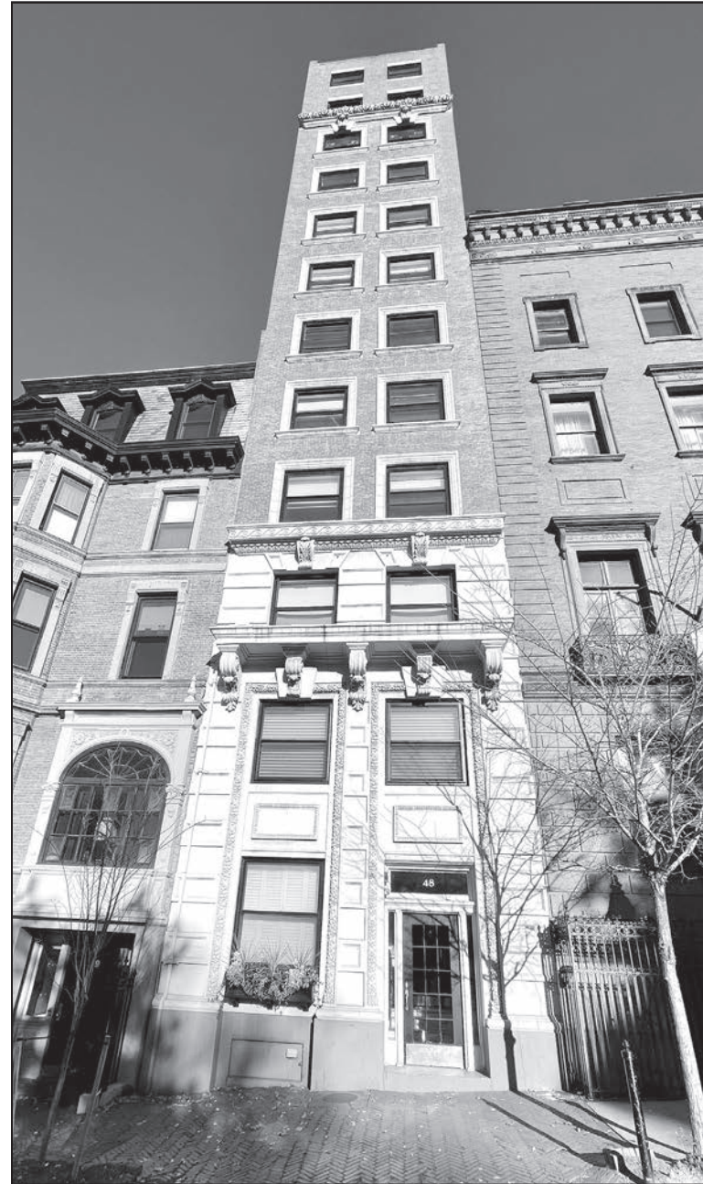
The masonry detail in the last clue is on 48 Beacon Street, built circa 1920. In city records, Architect Arthur H. Vinal is listed as the owner. Those early records have a violation we would not see today: operating an elevator without a licensed operator.
