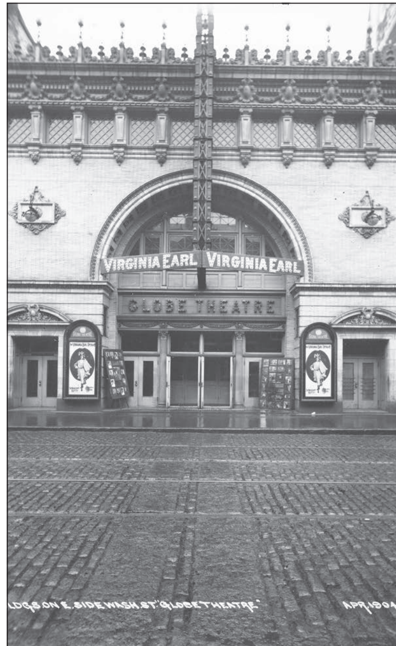
The ornamental plaque in the last clue is on the façade of the Empire Garden restaurant at 690 Washington Street. Architect Arthur H. Vinal designed this building. It was constructed in 1903 as the third version of the Globe Theater. Today's answer is a photo of the property from 1904.
