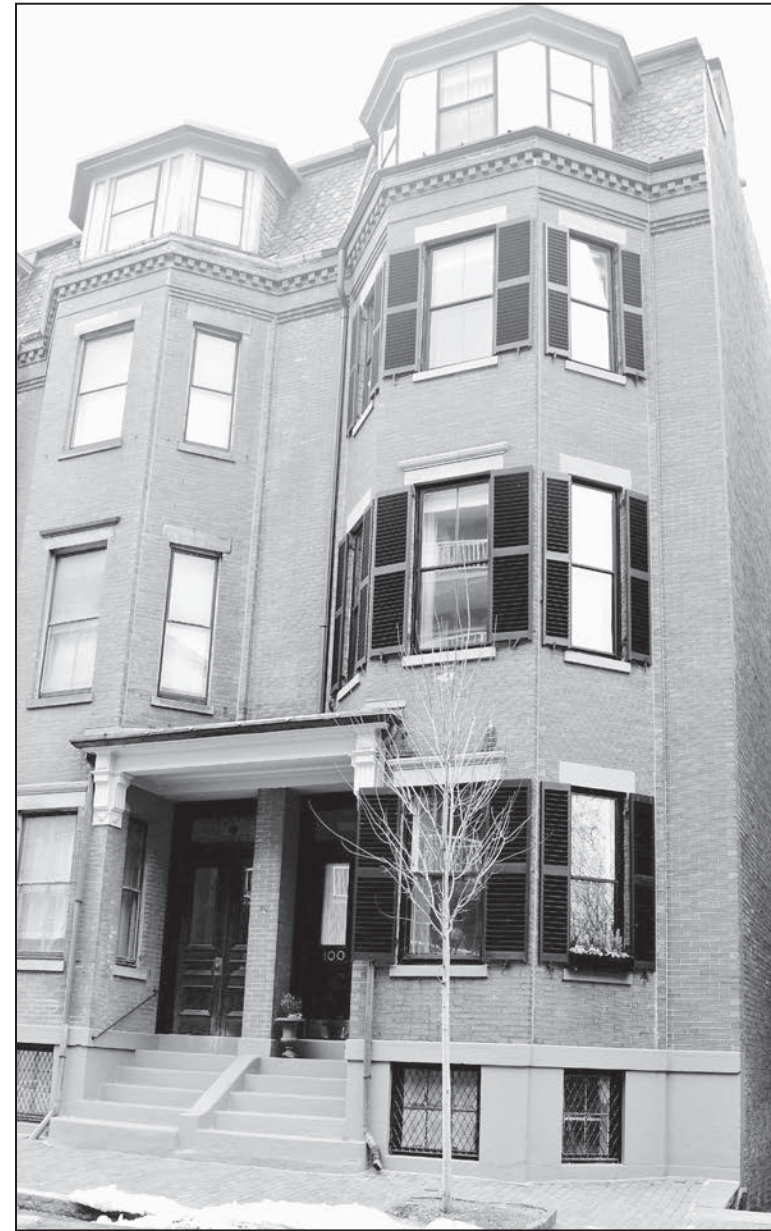
The dormer in the last clue is on 100 Pinckney Street, built circa 1890. French architect François Mansart is credited with popularizing the mansard roof named after him and the dormers he designed into that roof to bring light to attic bedrooms.
