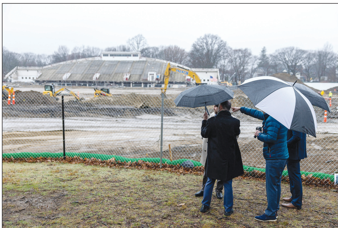
Demolition work is underway at White Stadium
